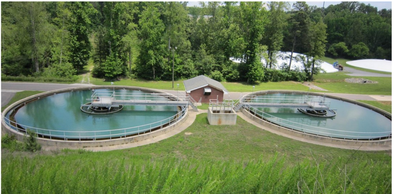
Water treatment site
